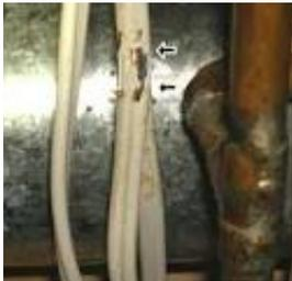
The problem with the “unseen” wiring in the walls **and the attic** where the rodents have been chewing, **you can't see the wiring**. If the insulation is chewed to where the bare copper would touch another bare wire in the cable, a short-circuit (high amperage) would occur and the circuit breaker or fuse is required to open the circuit immediately.
